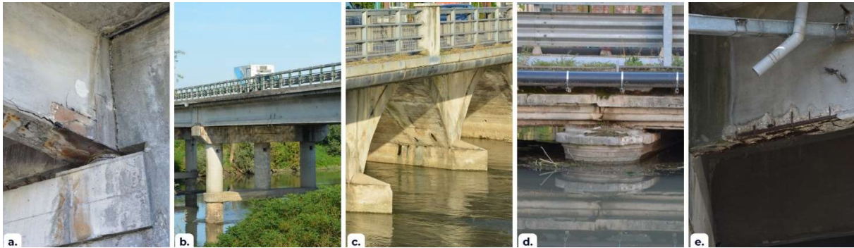
Figure 9: Defects registered during the survey of the route. The abutment (a) and piers (b) deterioration; Presence of active and passive humidity phenomena (c); the debris presence (d); Concrete loss and reinforcement oxidation (e)
