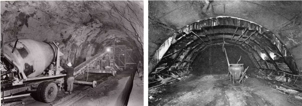
Figure 29: Use of conveyor belt for concrete casting (left) (courtesy Bertino E.), use of pneumatic impulse pump for concrete casting Tunnel of Petit Monde – Grasso (1969) (right)
