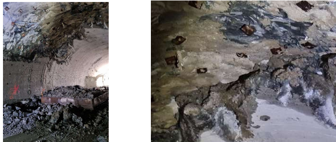
Figure 27: Picture of the rock bolts installed on the rock mass during excavation that were exposed after the demolition of the final concrete lining in Mont Blanc road tunnel
