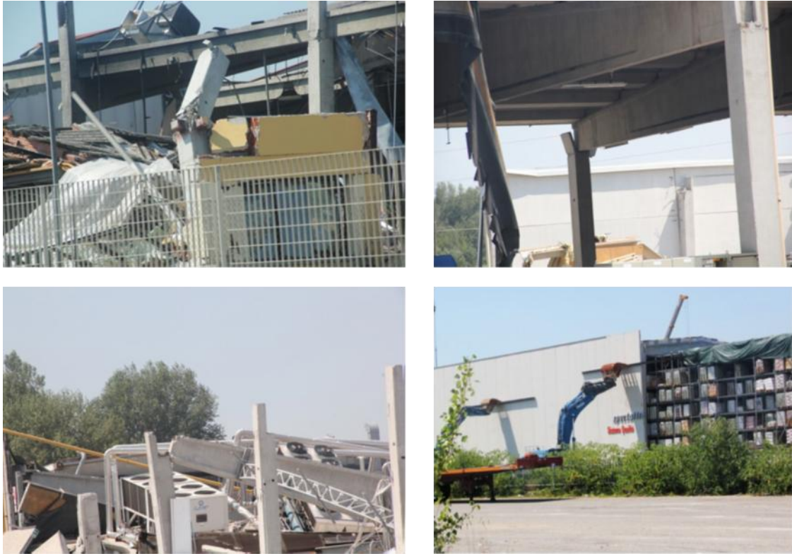
Figure 37. Some failures in industrial buildings, as reported in Bathalia et al. (2019): short column effect (top left); connection failure (top right); loss of support of beam (bottom left); vertical cladding panel collapse (bottom right).
