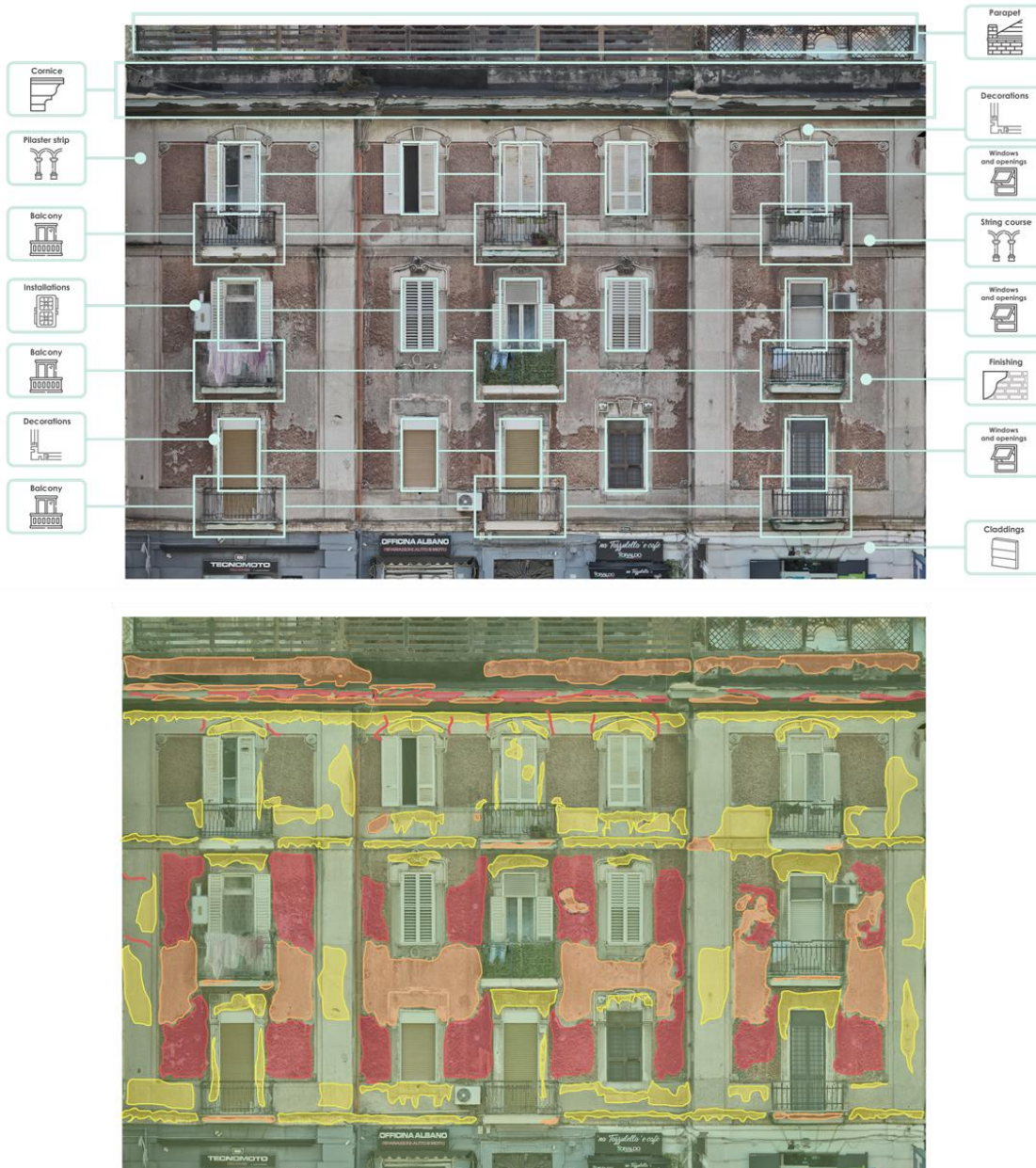
Figure 2. Facade analysis based on technological elements and degradation characterization
