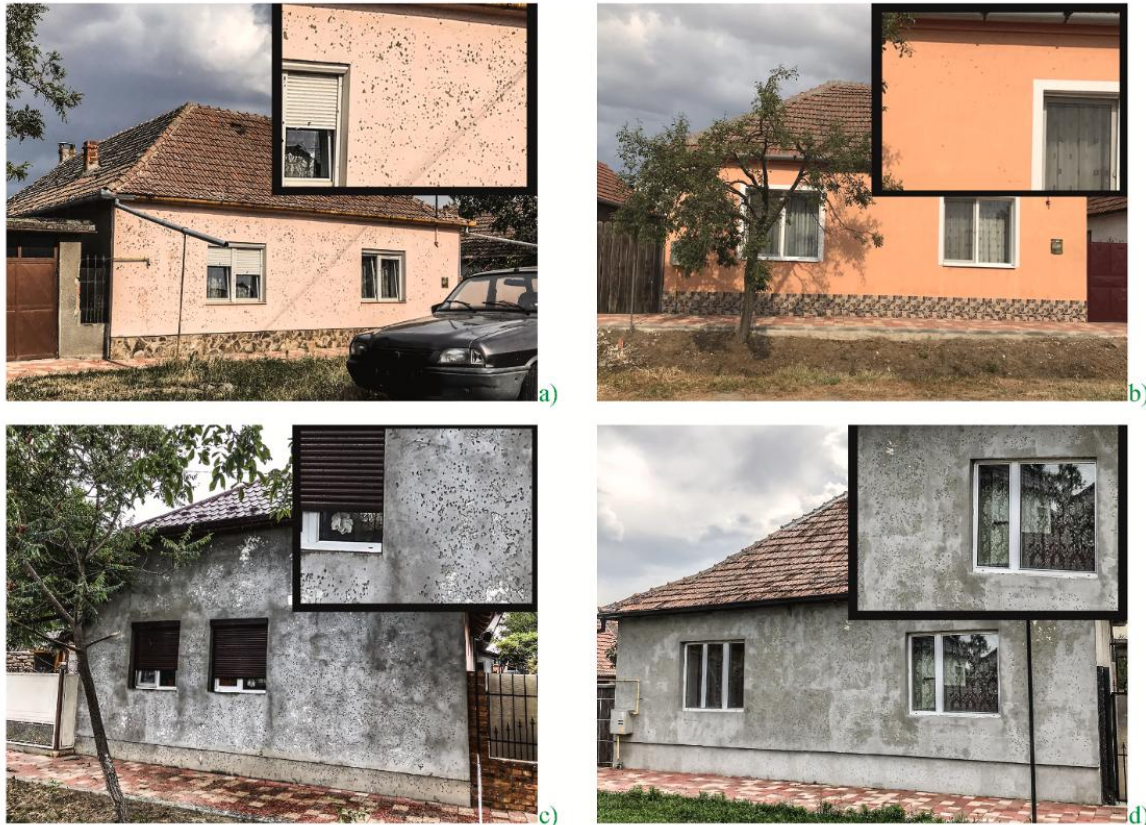
Figure 95. Hail-induced damage patterns: (a) Facade 1; (b) Facade 2; (c) Facade 3 and (d) Facade 4 (from Calotescu et al., 2024).
