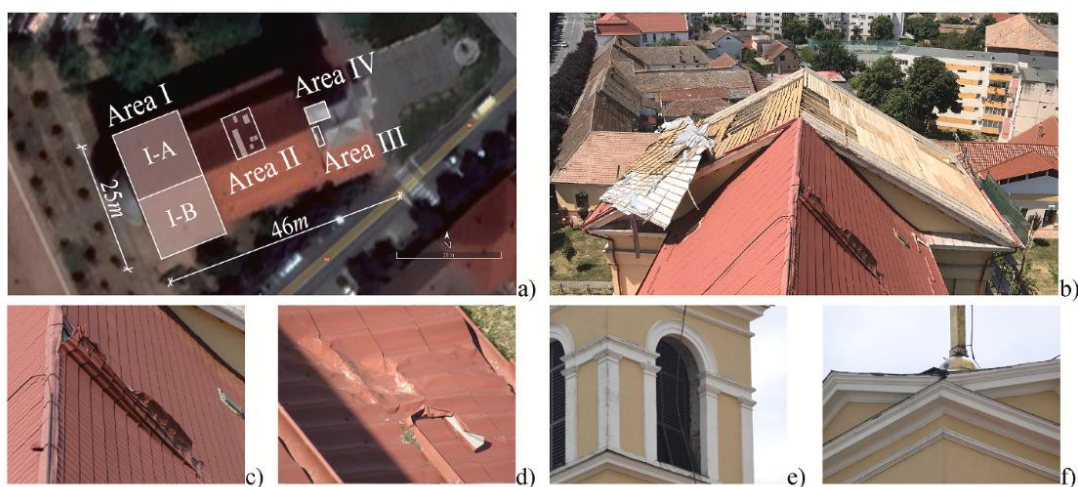
Figure 94. Wind-induced damage to Building A: (a) top view and damage areas; (b) roof damage in Area I (partially restored); (c–d) roof damage in Area II; (e) window damage in Area III; (f) roof damage in Area IV (from Calotescu et al., 2024).
