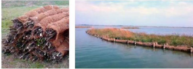
Figure 1. Examples of fascines produced locally (upper left) and then placed to protect salt marsh edges from erosion in LIFE VIMINE (Barausse et al., 2015)
