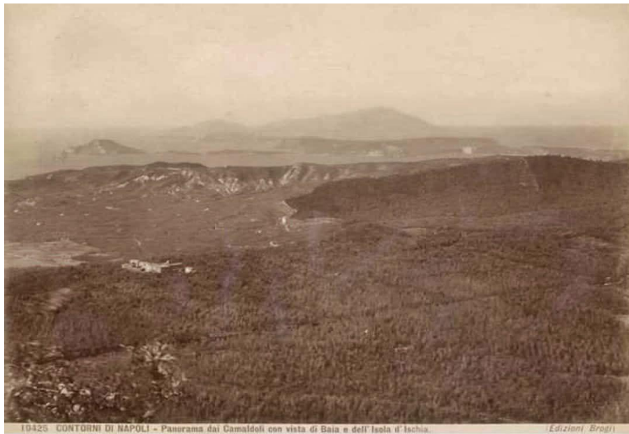
Figure 9: Soccavo and Pianura in the late XIXth Century, before the urbanisation process
