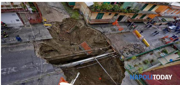
Figure 37: the via Campanile sinkhole in 2015, via napolitoday.it
