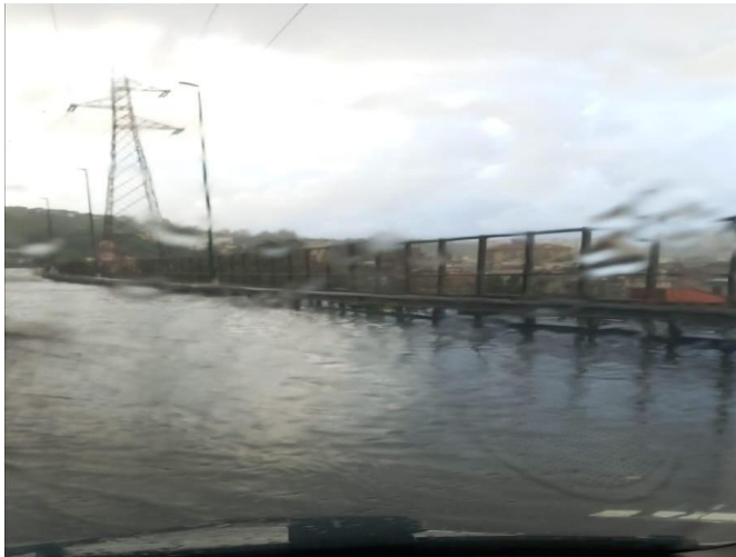
Figure 40: a flood at the Via Epomeo flyover, 2023.
