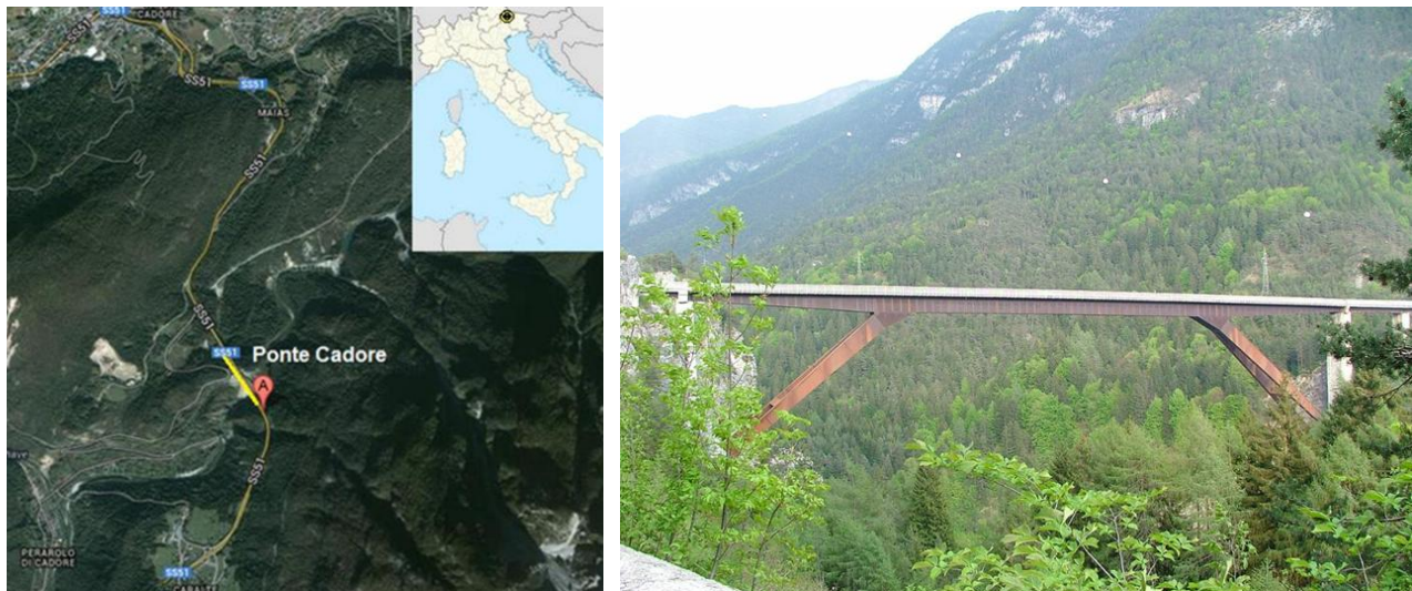
Figure 5.4-1 – Geolocalization and lateral view of the Cadore Bridge in Perarolo di Cadore (BL).
