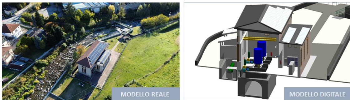
Figure 7: Meano hydroelectric power station in Pomaretto (TO) used as a case study
