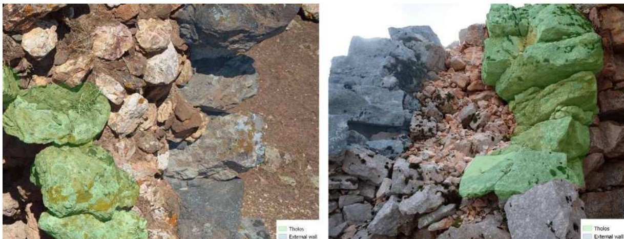
Figure 105. Backfill Material: (a) Soil and Stones of Various Sizes, in Nuraghe Sa Domu e' S'Orcu, Domusnovas (SU); (b) Stones, in Nuraghe Mereu, Orgosolo (NU).
