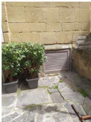
Figure 49. Points of possible ingress of floodwater and position of the main entrance above the road pavement.
