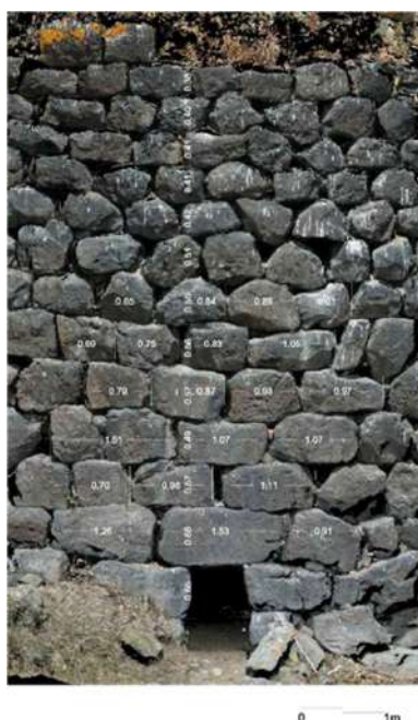
Figure 123. Detail of the masonry techniques.
