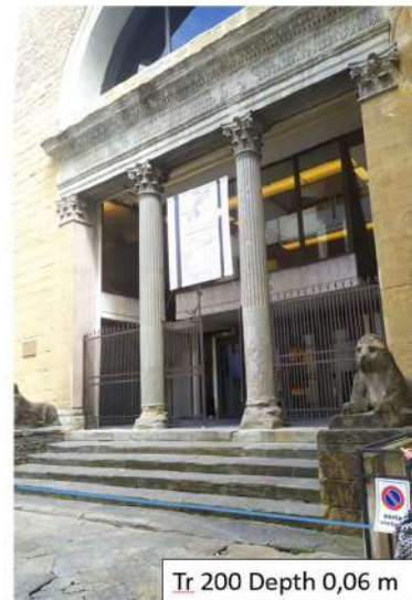
Figure 49. Points of possible ingress of floodwater and position of the main entrance above the road pavement.
