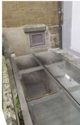
Figure 49. Points of possible ingress of floodwater and position of the main entrance above the road pavement.
