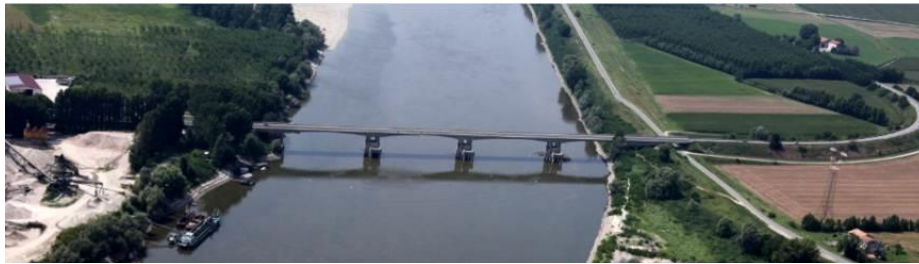
Figure 5-1 – San Benedetto Po bridge (East side).
