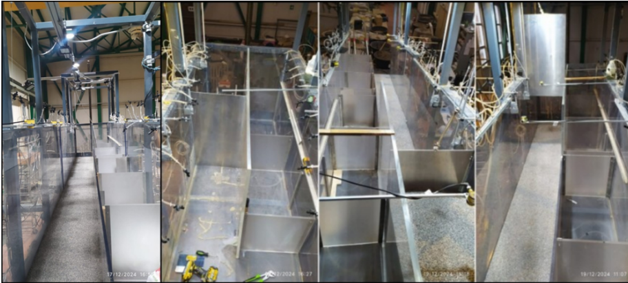
Figure 3. Picture showing the part of the original flume dedicated to the granular flow experiments (on the left) and details of the installation of the gate and opening system constituting the dam-break (centre and right).
