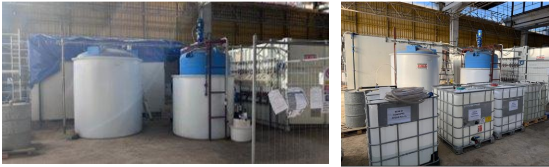
Figure 57: Pictures of EKRT Pilot Plant
