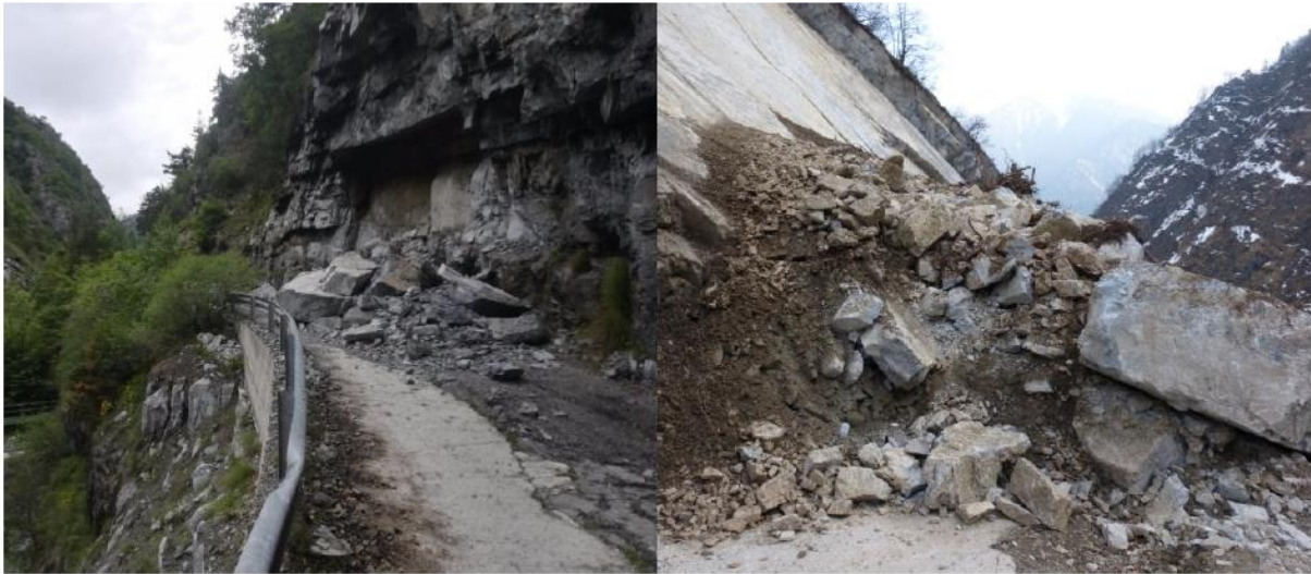
Figure 4. Instabilities of 2 June 2018 (about 250 m 3 ) and 25 February 2015 (more than 2000 m 3 ).
